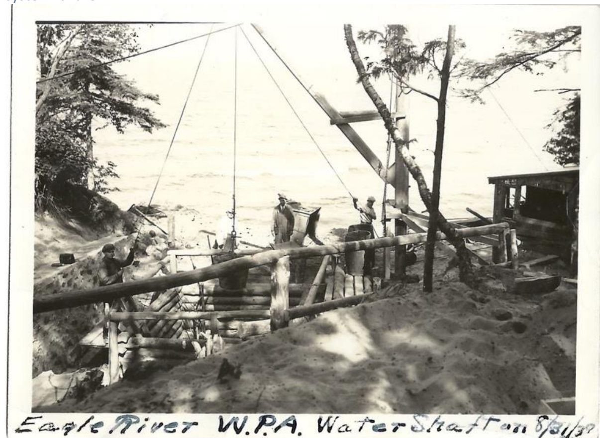
CONSTRUCTION OF THE DRINKING WATER SOURCE SHAFT IN 1939
